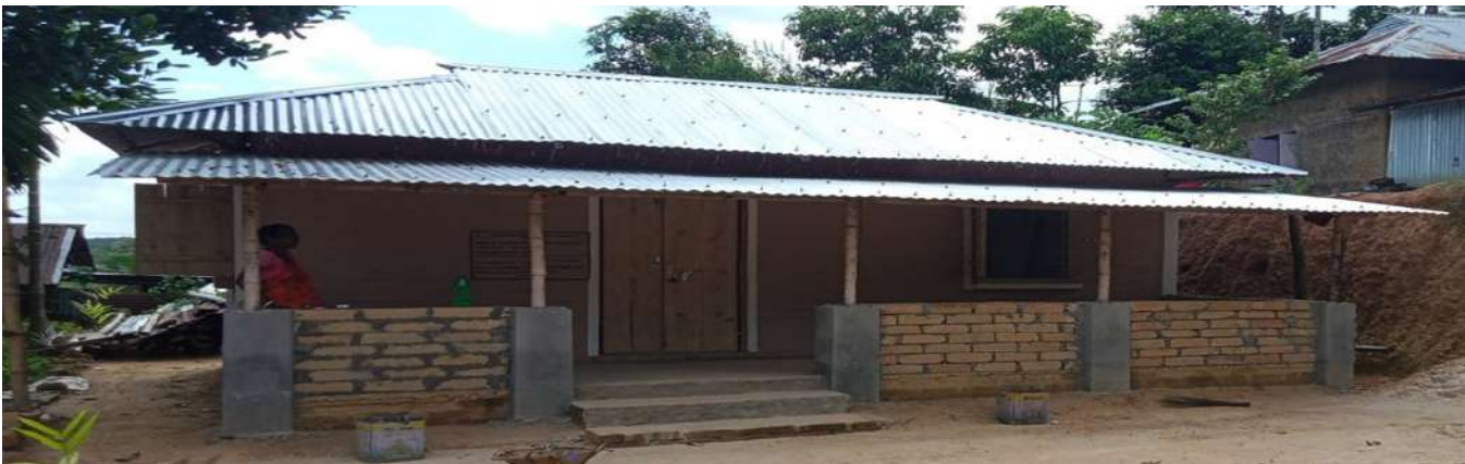
Training of SHG member for construction of stabilized mud block
