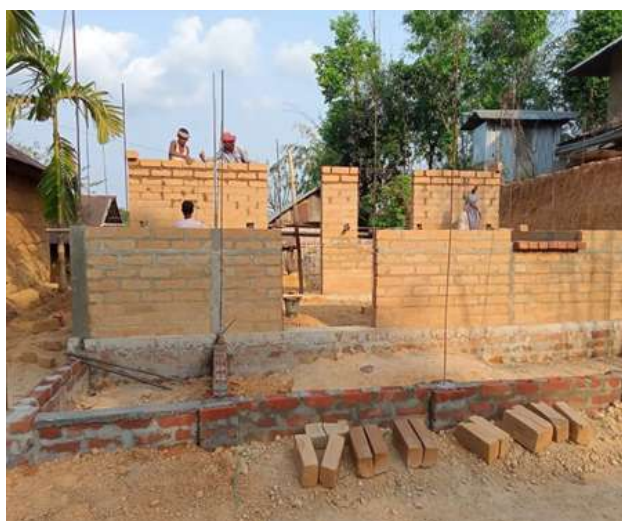
Stabilized mud block house of Smt Archana Dey under construction
