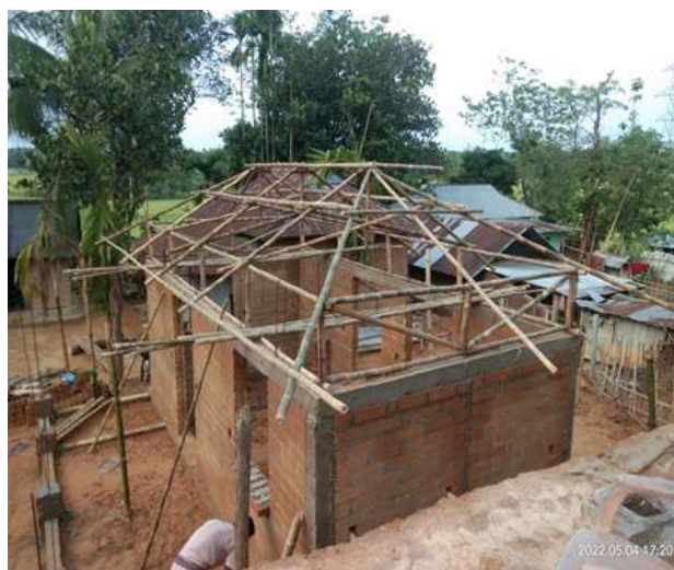
Stabilized mud block house of Smt Archana Dey under construction
