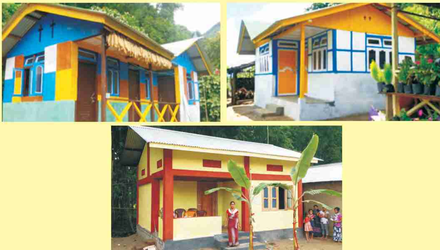
Pic. 5: Construction of houses under PMAY-G as per identified house design typologies
