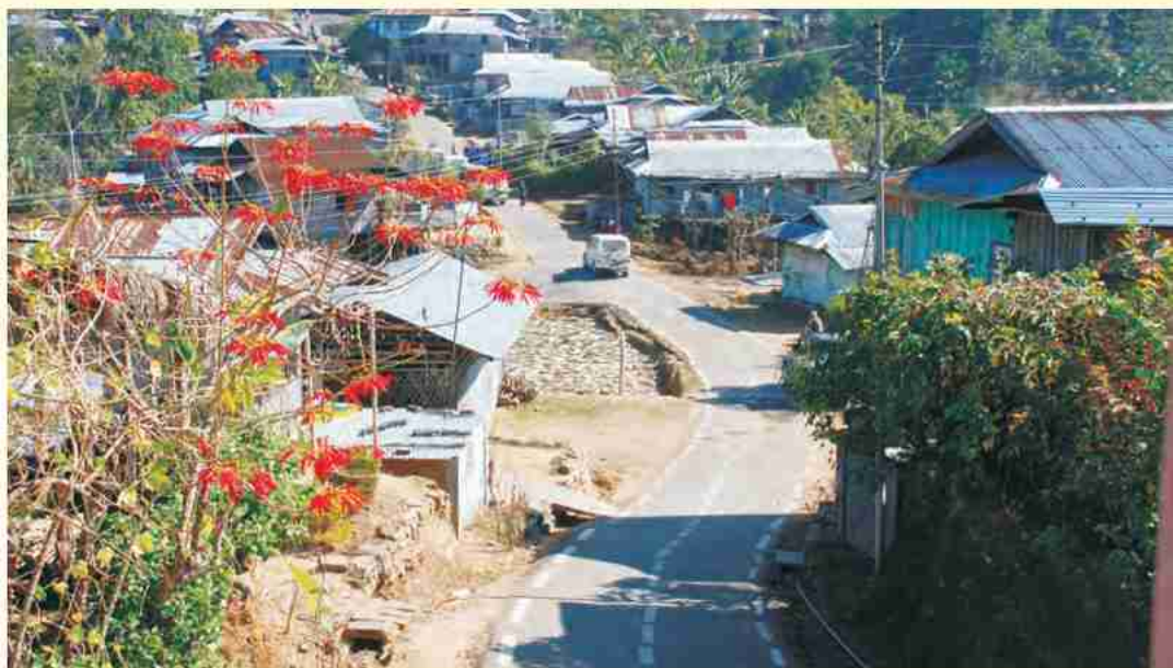
Water harvesting Tank in cluster - MGNREGA, Village-Yaongyimsen, Block-Changtongya, Distt -Mockokchong, Nagaland
