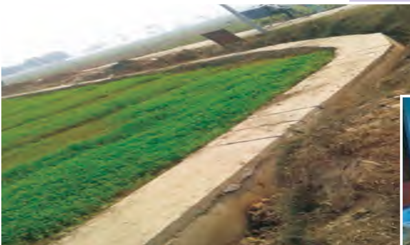
Pucca drain system in Dasna cluster, Ghaziabad, Uttar Pradesh.
