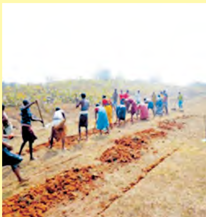
Water Absorption Trench IWMP-1 (2009-10) Project, Block- Saharapada, District-Keonjhar, Odisha Latitude-21.77551, Longitude- 85.86762
