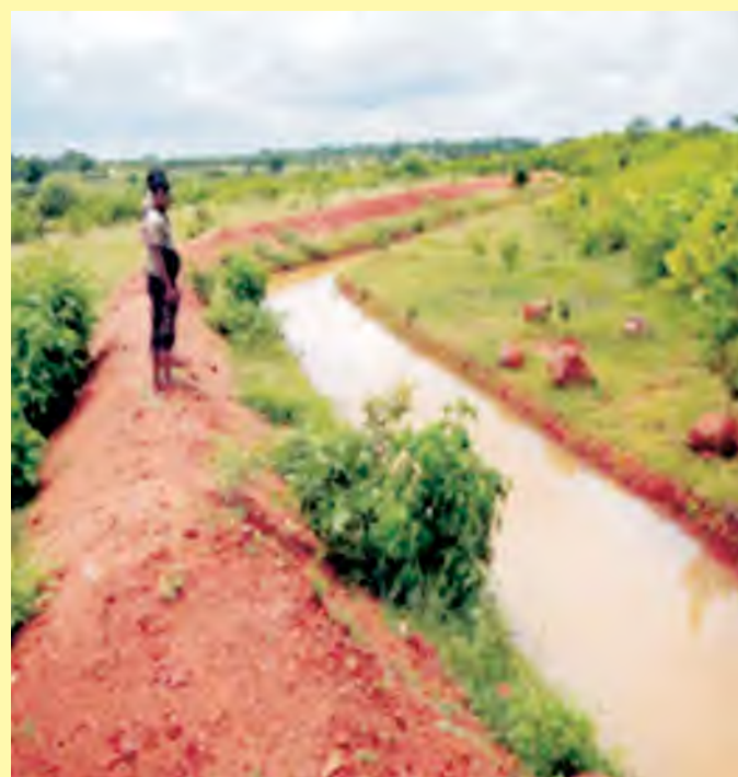
Water Absorption Trench IWMP-1 (2009-10) Project, Block- Saharapada, District-Keonjhar, Odisha Latitude-21.77551, Longitude- 85.86762
