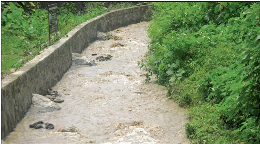
Protection wall built under MGNREGA in Manipur
