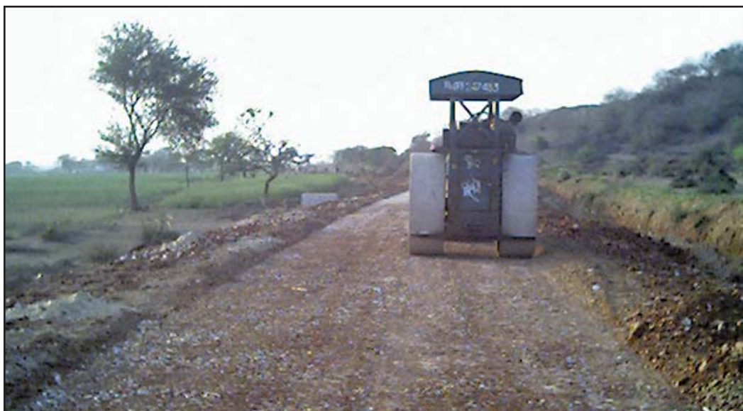
PMGSY road under construction in Andhra Pradesh
