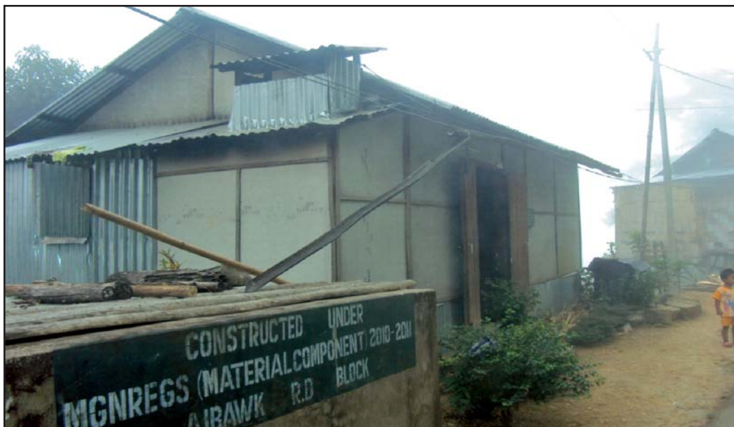
House constructed under IAY. The rain water is trapped through a channel made of bamboo connected to a water tank. The water tank is constructed under MGNREGA works in Mizoram
