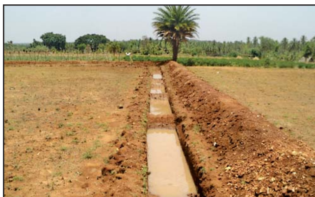
Trench cum pit Bunding under IWMP-8/2011-12, Taluk-Chennarayapatna, District-Hassan, Karnataka, Lat. & Long. -16°44'11.7" N 76°27'39" E
