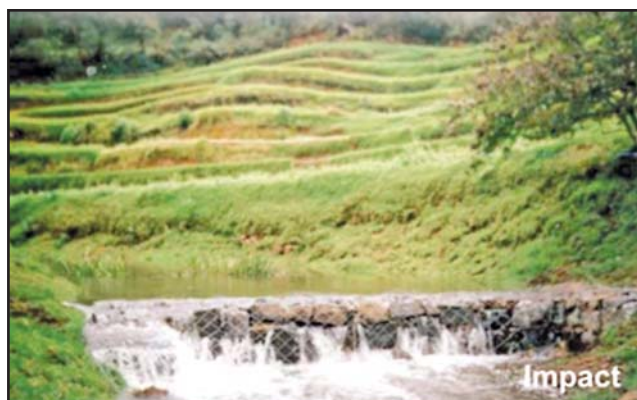
Construction of Gabion Checkdam under DPAP-XII Batch in Mannavanur Watershed of Kodaikanal Block in Dindigul District of Tamil Nadu
