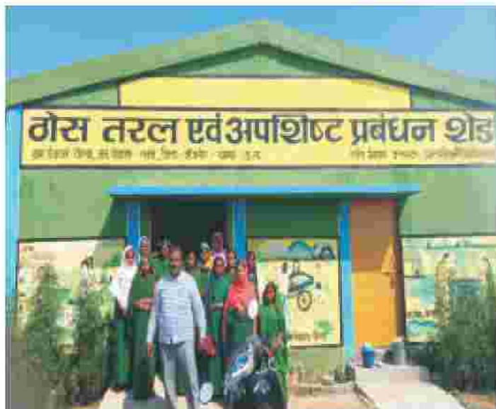
Solid Waste Management Shed, Jetha cluster, Janjgir Champa Dist., Chhattisgarh
