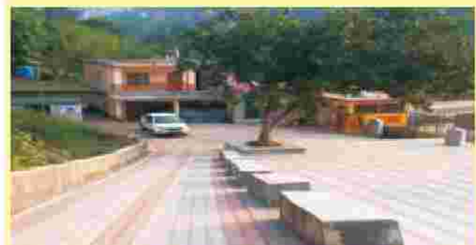
Paved Road at Deoli Gram Panchayat, Himachal Pradesh, Bilaspur District, Himachal Pradesh
