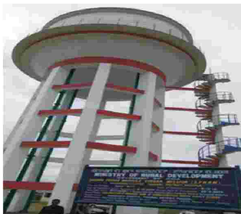
Overhead Water Tank in Khangabok cluster, Thoubal District, Manipur
