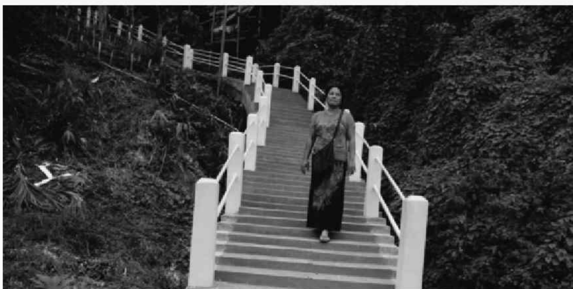
Construction of Foot Steps under MGNREGA
