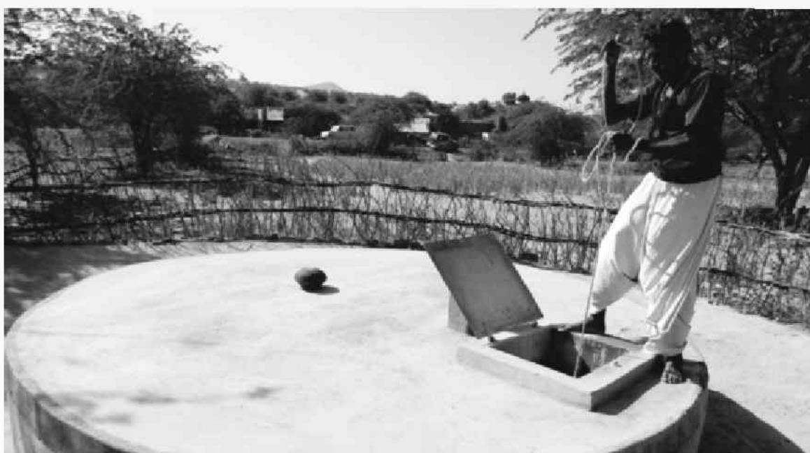
Tanka (well) Construction under MGNREGA, Distt.-Badmer, Rajasthan
