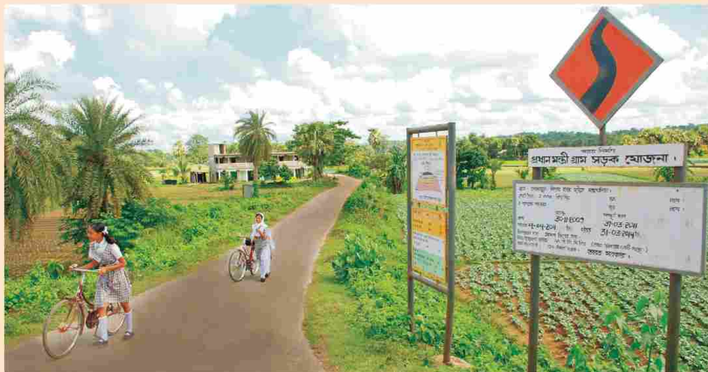
PMGSY Road Nidoya to Marjunia, Vill. Bhesimara, Block Kathalia, Distt. Sepahijala, Tripura
