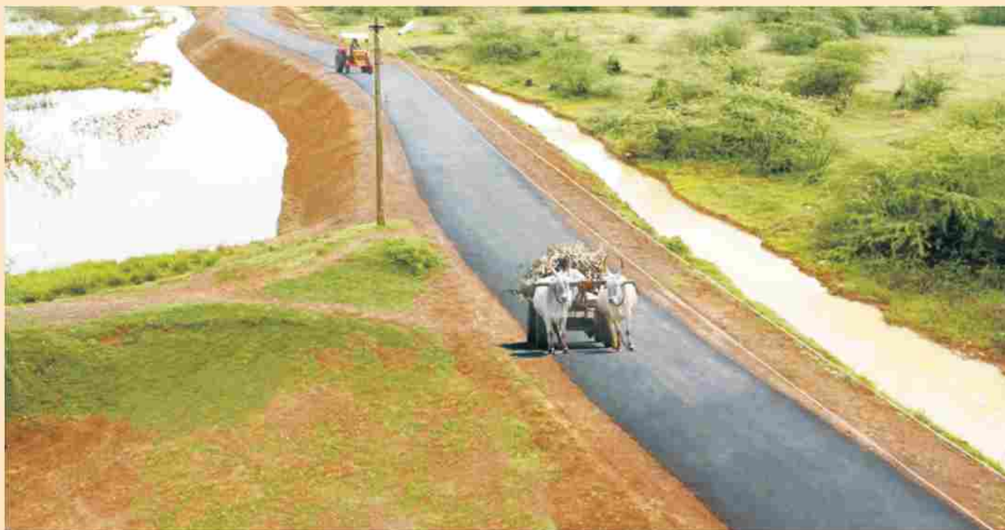
PMGSY road, Distt. Kanchheepuram, Tamilnadu
