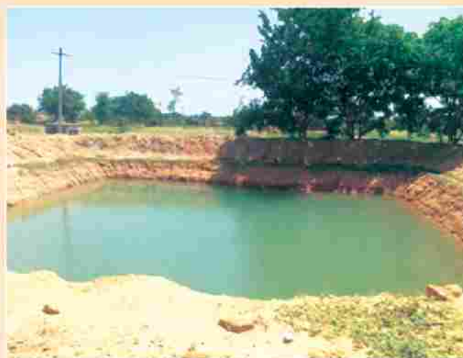
Farm pond construction
