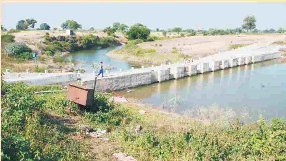
Stop Dam & Culvert under MGNREGA, Madhya Pradesh
