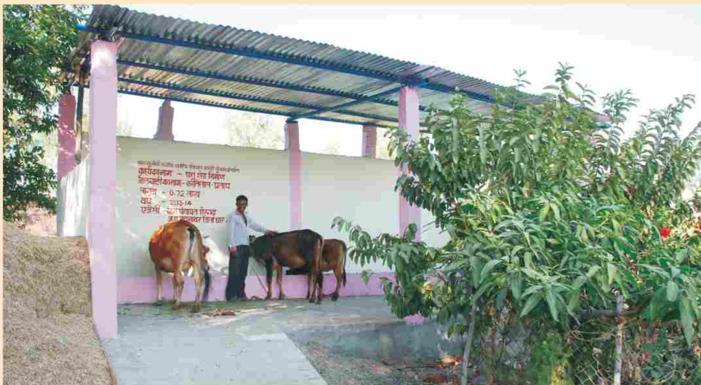
Cattle Shed under MGNREGA, Madhya Pradesh
