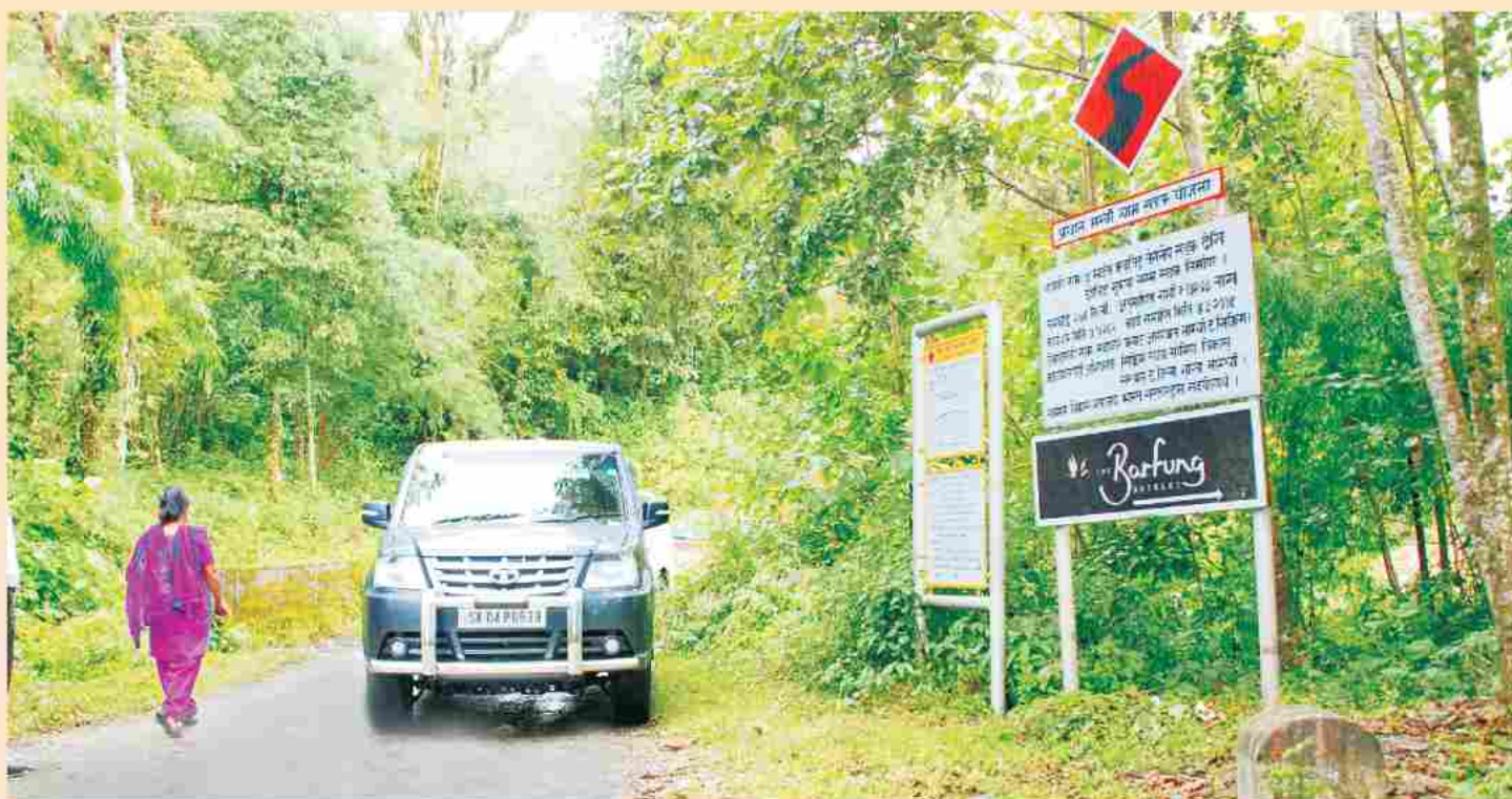
PMGSY road, Block Ravangla, Distt. South Sikkim
