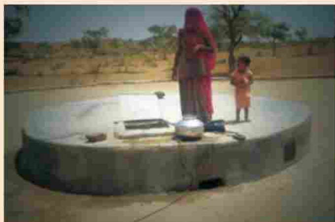
Tanka Construction at primary School Aklavyanagar
