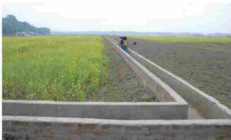
Irrigation Channel-MGNREGA, Vill. Buraburi, G.P. Buraburi, Block Mayong, Disstt. Mori Gaon, Assam
