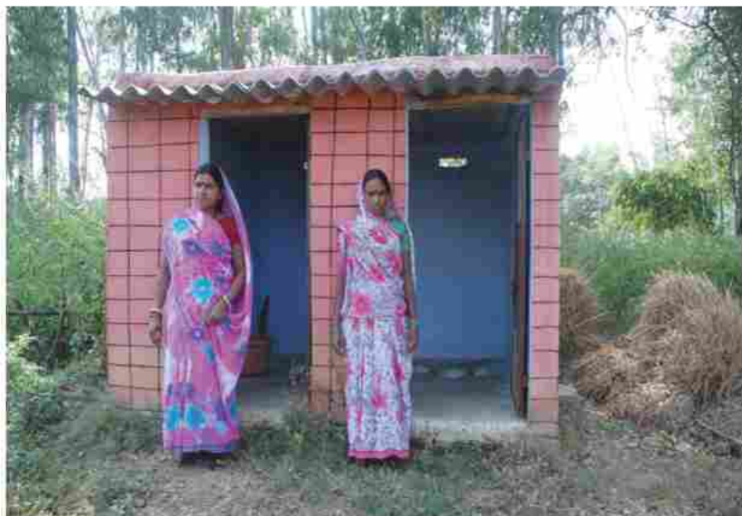
Construction of Latrin - MGNREGA & NBA, Vill. Revnadih, G.P. Herodih, Block Jainagar, Distt. Kodarma, Jharkhand
