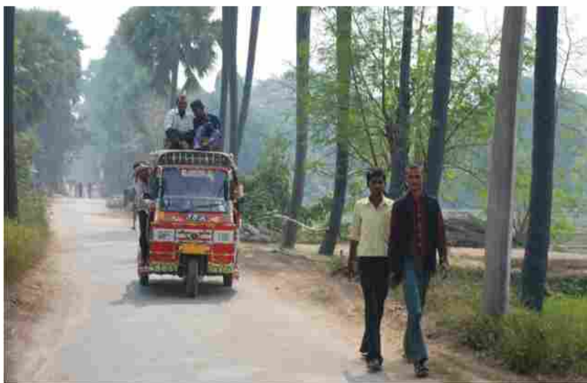
PMGSY Road, Vill. Sadipura, Distt. Navada, Bihar
