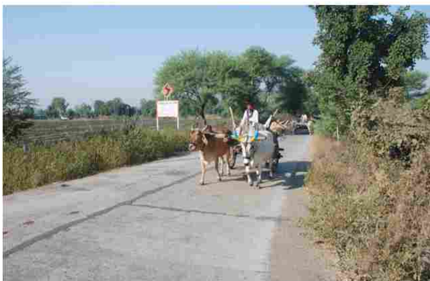
PMGSY Road (NH 3 to Chatha), Vill. Chamari, G.P. Moia, Block Baiora, Distt. Rajgarh, M.P.
