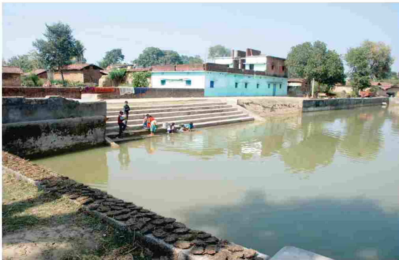
Renovation of Pond & Guard Wall under MGNREGA Vill. Ratan Pur, G.P. Barka Khurd, Block Ichak, Distt. Hazaribagh, Jharkhand
