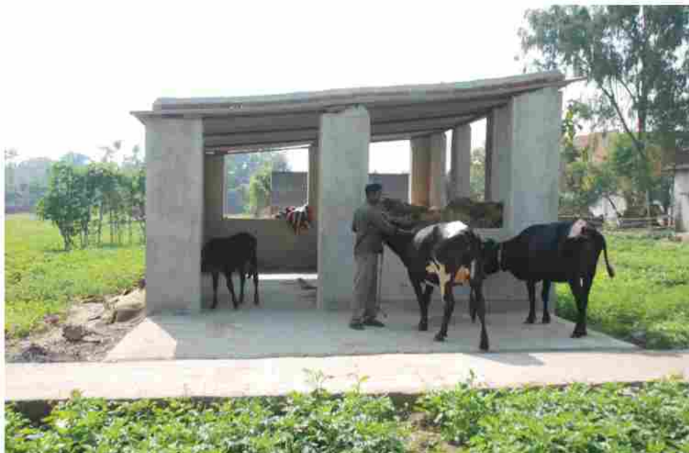
Cattle Shed - MGNREGA Vill. Hirodih, G.P. Herodih, Block Jainagar, Distt. Kodarma, Jharkhand
