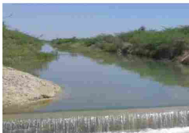
Improving water availability through rainwater harvesting by constructing checkdam
