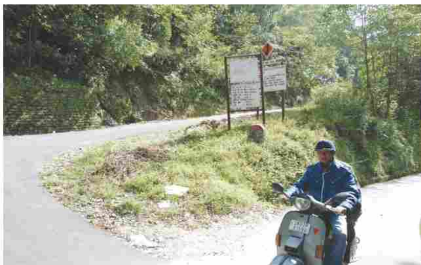
PMGSY Road, Mile Kewzing Legship road to Mamrung Gump, Block Ravangla, Distt. South Sikkim
