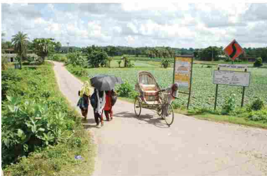
PMGSY Road Nidoya to Marjunia, Vill. Bhesimara, Bloack Kathalia Tripura
