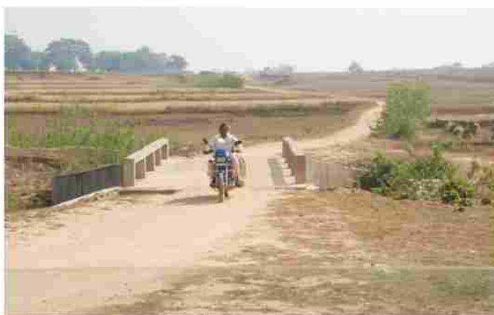
Culvert - MGNREGA, Village Gunja, G.P. Kurha, Block Ichak, Distt. Hazaribagh, Jharkhand
