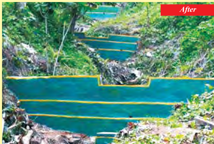
IWMP – IX / 2012-2013, Thodupuzha Block, Idukki – Bund construction with Coir Geo Textiles
