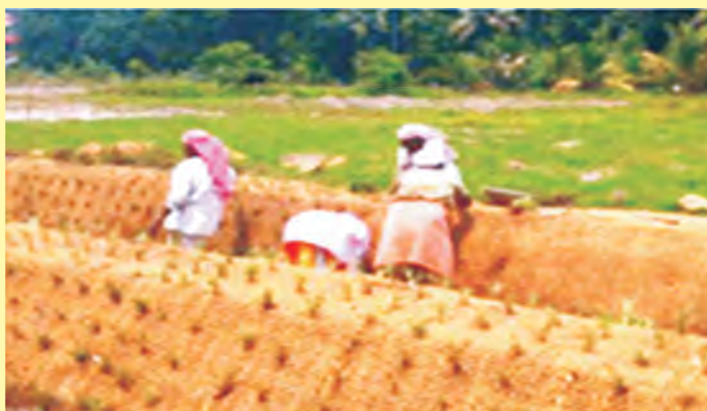
IWMP – IX / 2012-2013, Thodupuzha Block, Idukki – Bund construction with Coir Geo Textiles
