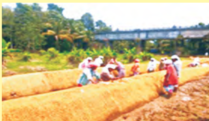
IWMP – IX / 2012-2013, Thodupuzha Block, Idukki – Bund construction with Coir Geo Textiles
